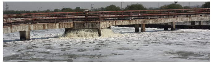
Fig. 6. Aeration Treatment Plant
